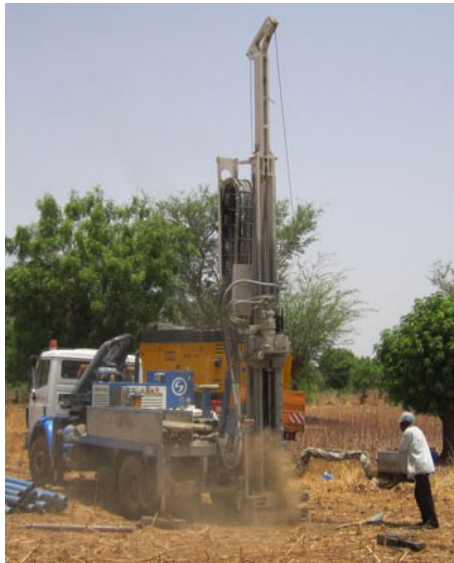
Brunnenbohrung in Godola-Hosséré
